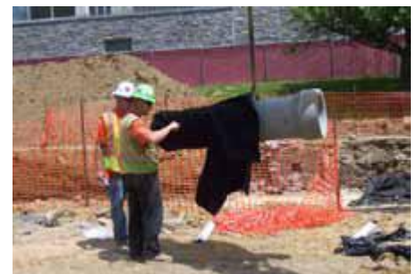
Fig. 14 Seal the pipe boot with band clamps and duct tape.
