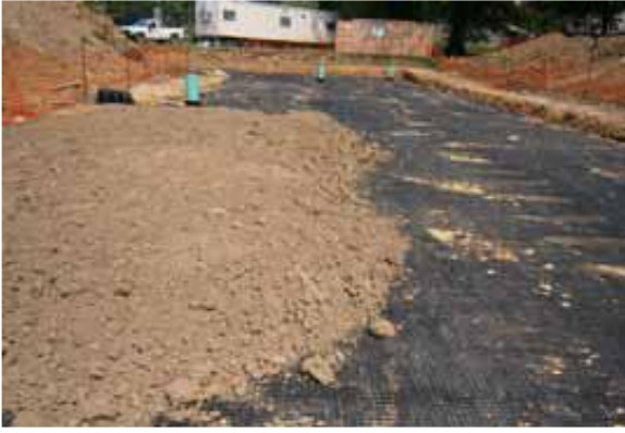
Fig. 19 Pushing backfill parallel to the Geogrid.
