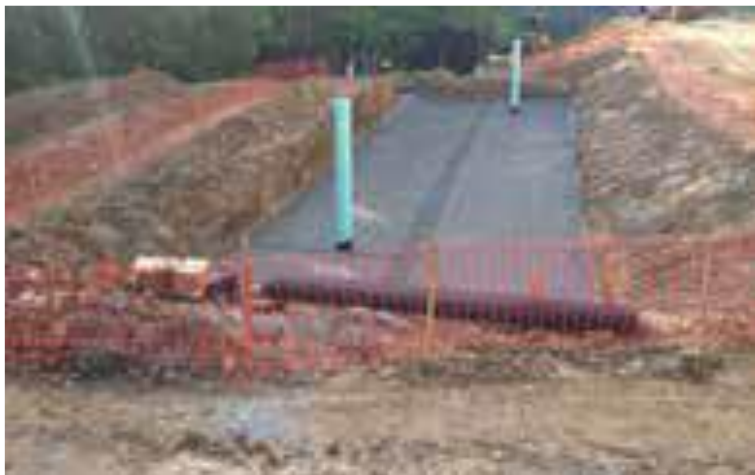
Fig. 20 Secure the installation with temporary fencing.
