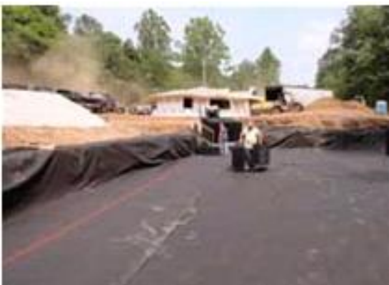
Fig 10: Use a String line & marking paint to square the system footprint.
