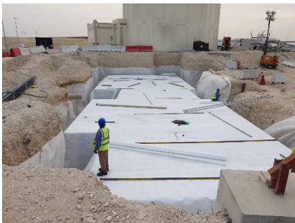
Fig. 12 Encapsulate STORMVAULT Tanks with geotextile
