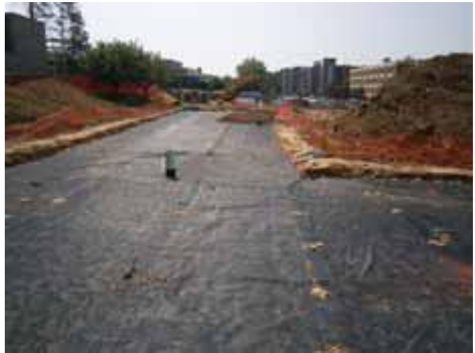
Fig. 18 Overlap Geogrid 18" (300mm) or as required by plans.
