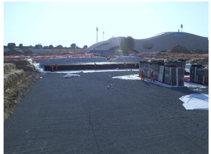
Fig. 7 & 7A Base must be smooth to ensure units fit together without gaps.
