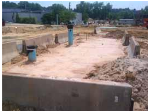
Fig. 21 Secured STORMVAULT Tank installation using Jersey Barriers.
