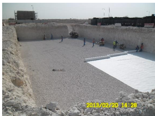
Fig 8: Overlap Geotextile by minimal 12" (300mm) or more. Pull Wrinkles out of Geotextile
