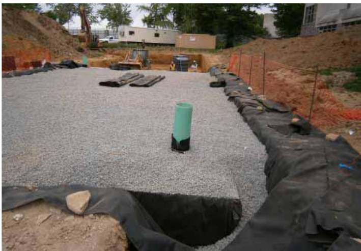
Fig. 17 Use an LGP dozer to push backfill over STORMVAULT Tank units.
