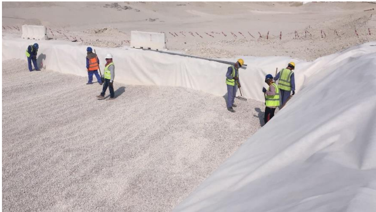
Fig. 7 & 7A Base must be smooth to ensure units fit together without gaps.
