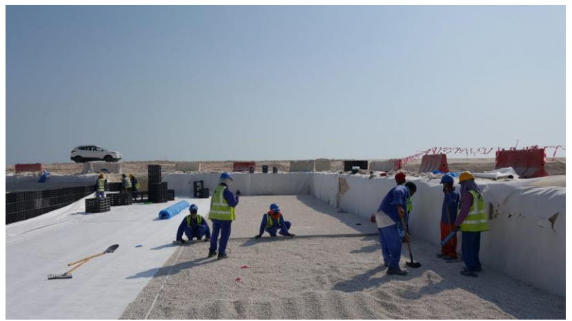
Fig. 3 Compacted and Levelled subbase to 95% proctor
